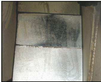
Chute liner using spacer under trailing edge.
