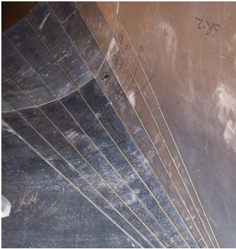
Multiple CRODON sections cut and welded for liner in limestone hopper.
